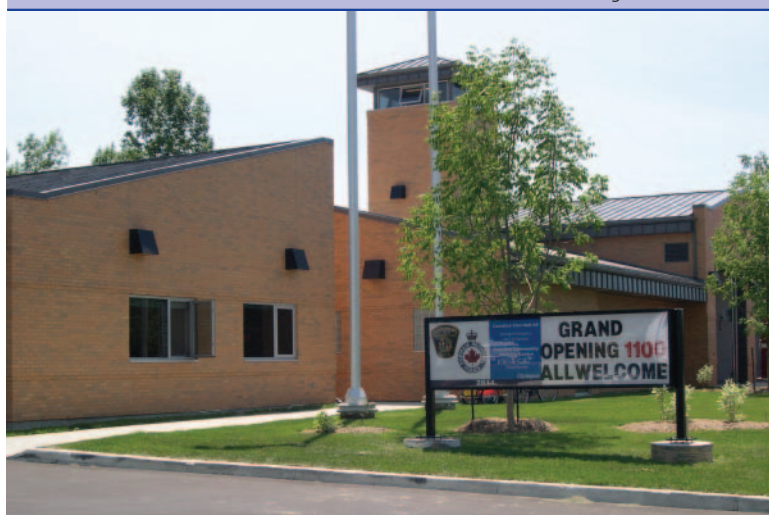
Clarington Fire Hall office
