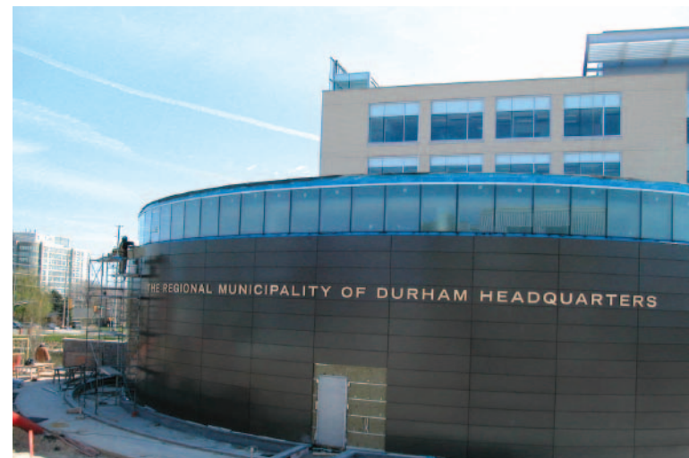
Regional HQ under construction in May of 2005
