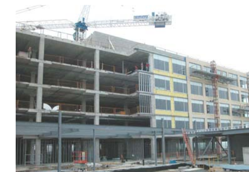
The Regional Headquarters under construction May 2004.
