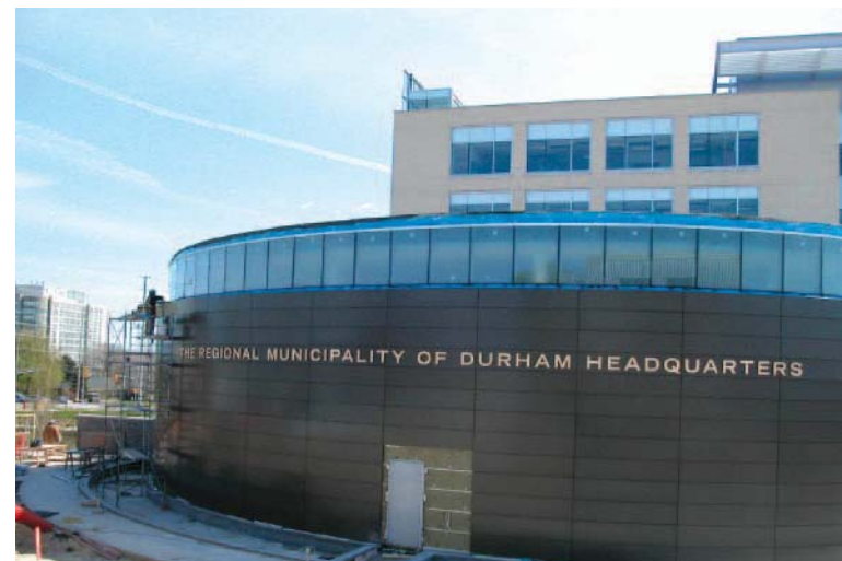
Regional HQ under construction in May of 2005
