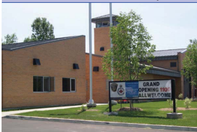
Clarington Fire Hall office
