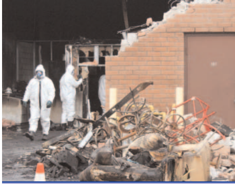
An explosion led to the discovery of a multi-million dollar methamphetamine lab after a fire in a Pickering industrial unit. See Page 8 for more details.
