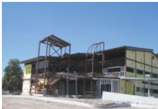
The new Whitby CPO under construction, June 2003.
