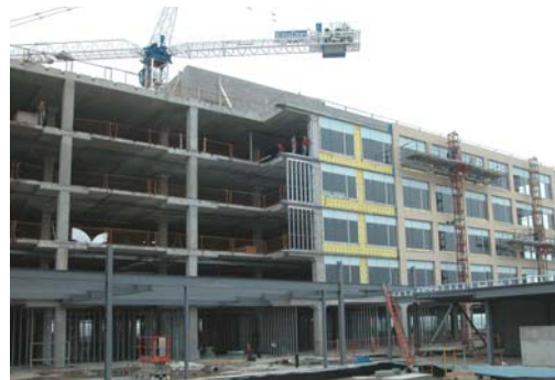
The Regional Headquarters under construction May 2004.
